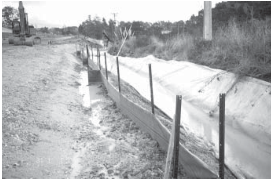
Silt Fence Installation on the ALPUR Motorway Project
