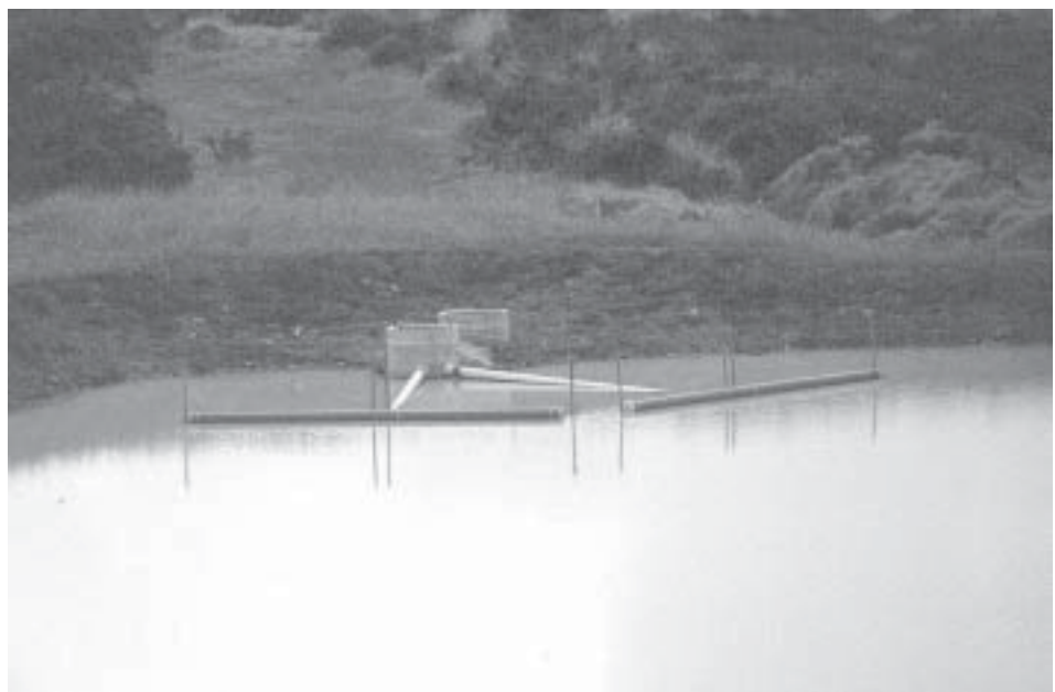
Typical Sediment Pond with a Decant System
